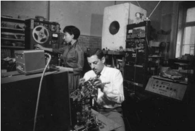
Plate 3.2 Louis and Bebe Barron in their Greenwich Village electronic music studio, 1956. The studio was equipped to record electronic sounds onto magnetic tape and synchronize them to motion picture images using 16 mm magnetic film recorders. (Bebe Barron)
