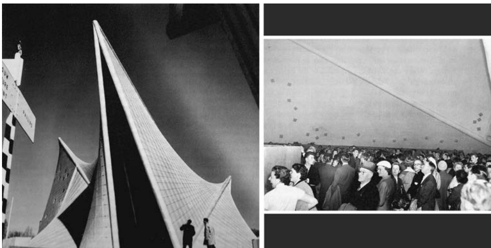
Plate 14.3 Exterior and interior of the Philips Pavilion at the Brussels World's Fair, 1958. Inside the pavilion, hundreds of small loudspeakers were mounted on the walls to create a moving path of sound. (Philips International BV, Eindhoven)
