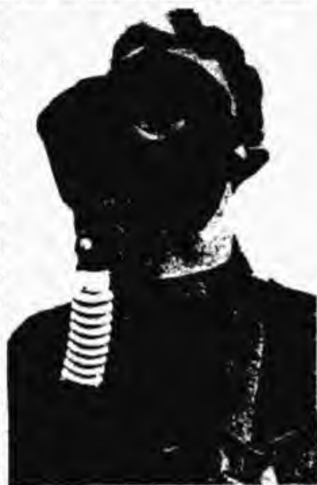
FIG. 111.—British Small Box Respirator.
