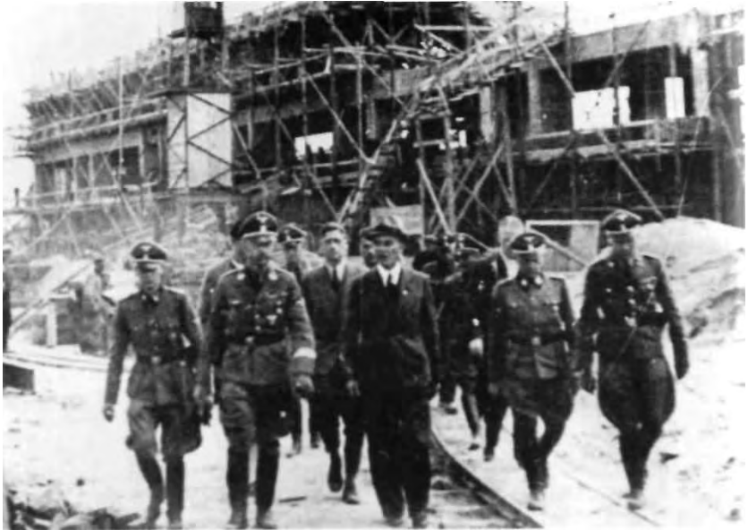
27. Inspecting IG Farben's Auschwitz, building site: Heinrich Himmler (second from left), foreman, Max Faust (site manager) and Rudolf Hoess (far right), July 1942.
