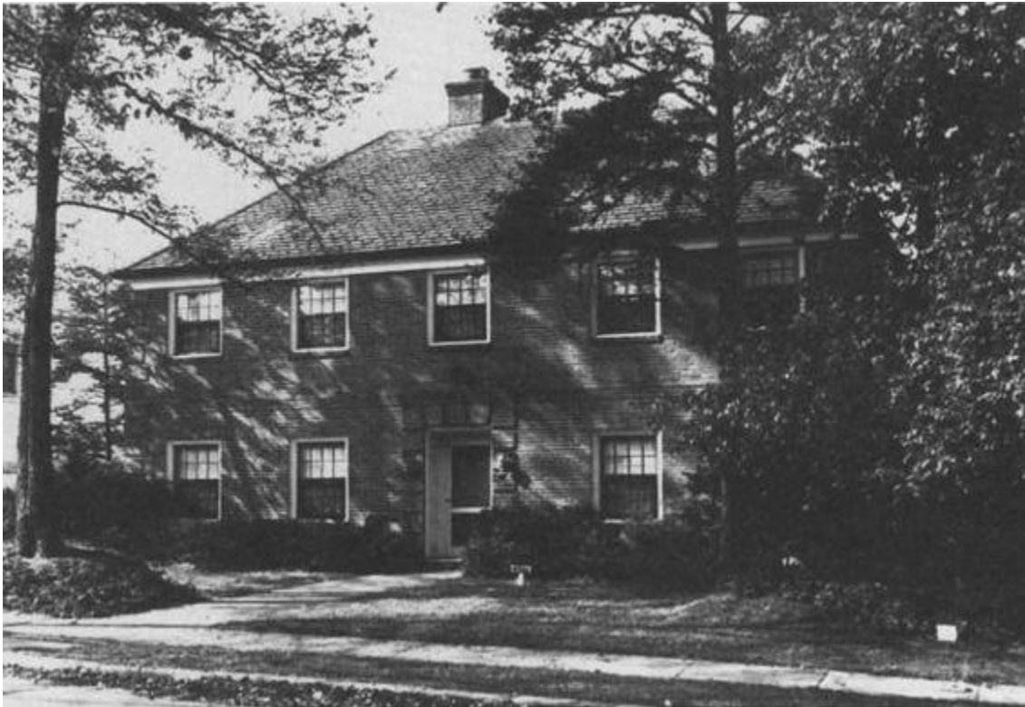
4936 Thirtieth Place NW, Washington, D.C., J. Edgar Hoover's home from 1938 until his death in 1972. Improvements and maintenance of the residence were paid for by the taxpayers. National Archives 65-H-1989-1.
