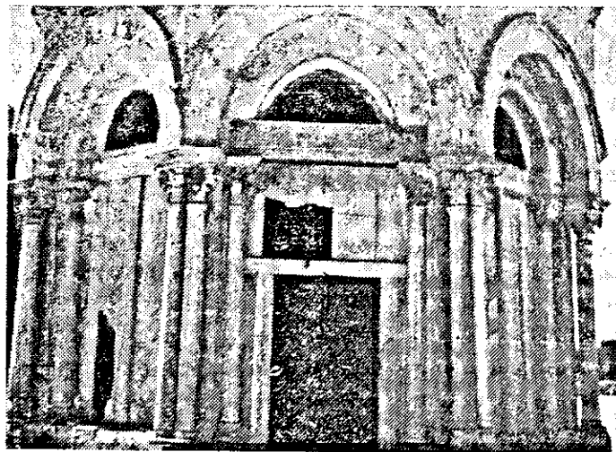
The damaged Sanctuary-Aksa Mosque.
